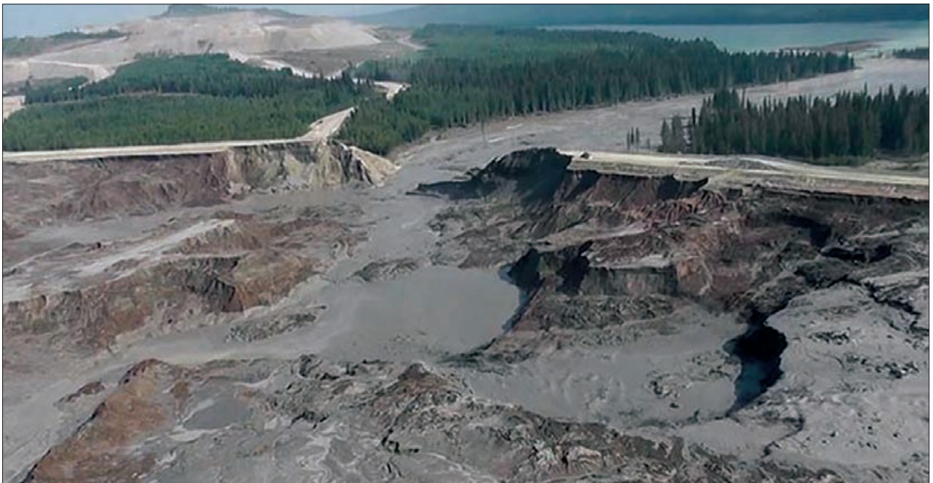
Tailing dam failure. Photo courtesy Synspecive ●●●
