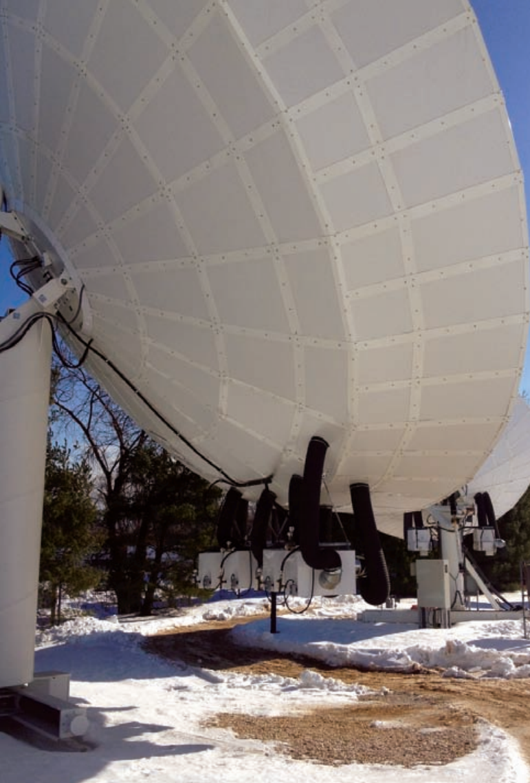
Plenum enclosure where gas heaters are installed. Photo courtesy Walton De-Ice ●●●
