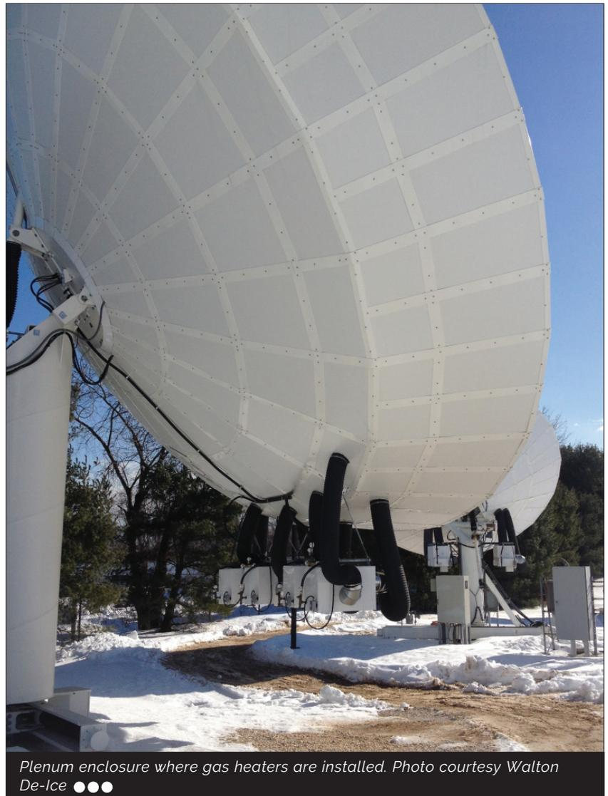
Plenum enclosure where gas heaters are installed. Photo courtesy Walton De-Ice ●●●
